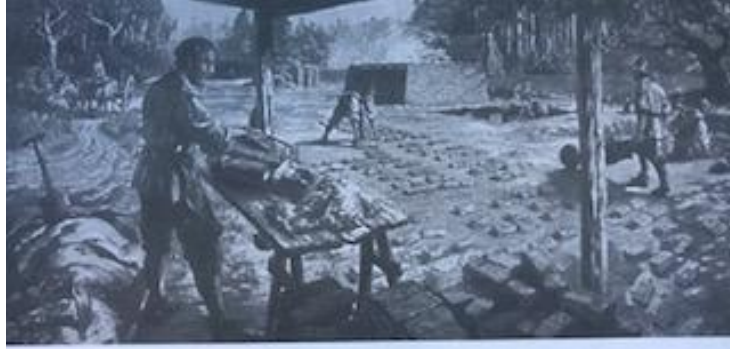
Above: Building permanent homes at Jamestown required bricks, which had to be molded by hand and baked in ovens.
